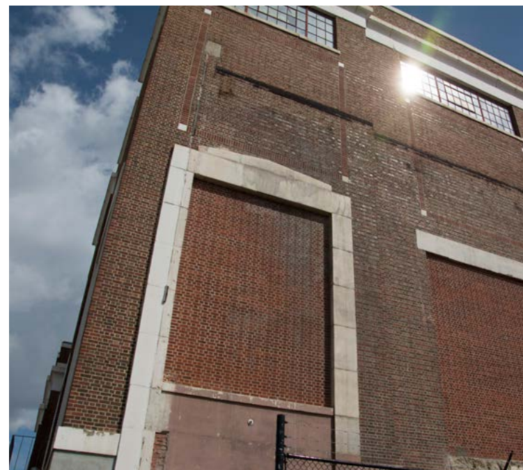
Rossdale Generating Station.
