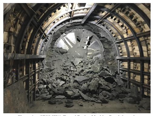
Figure 1e – SESS SW4, Tunnel Boring Machine Breakthrough
