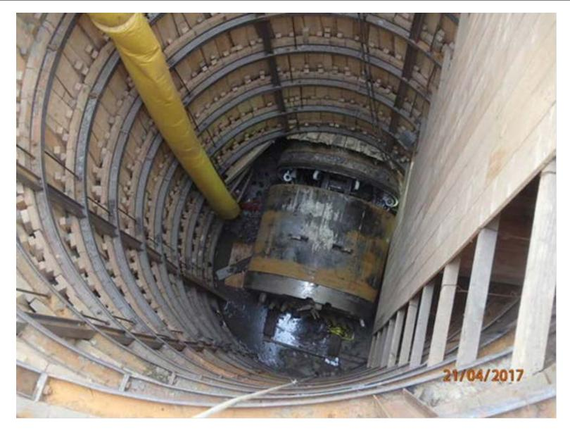
Figure 1a – NEST NC2/NC3, TBM at the Removal Shaft
