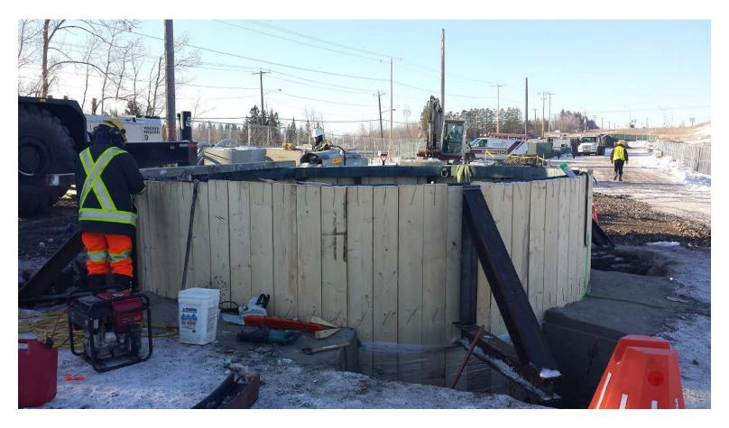
Figure 1d – SESS SW4 Working Shaft
