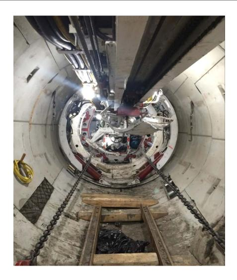
Figure 1d: NEST Stage NC2/NC3- Back end of the M100 TBM with a section of completed tunnel
