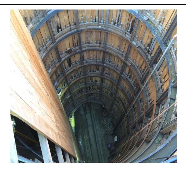
Figure 1h: SESS Stage SW4- 16'-6" diameter Working Shaft, depth of 18.0 m below ground elevation
