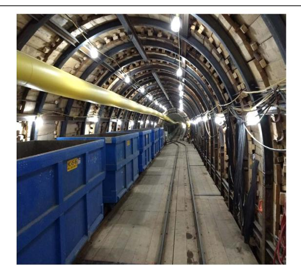
Figure 1e: SESS Stage SW4- Tunnel undercut, total length of 32 m, dirt cars on rail switch set-up
