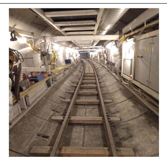
Figure 1f: SESS Stage SW4-TBM M126 Gantry & Trailing Shield- Tools, electrical equipment, ventilation, and all hydraulic components
