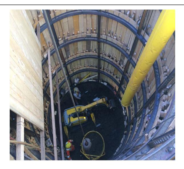
Figure 1a: NEST Stage NC2/NC3- Excavation of the main working shaft
