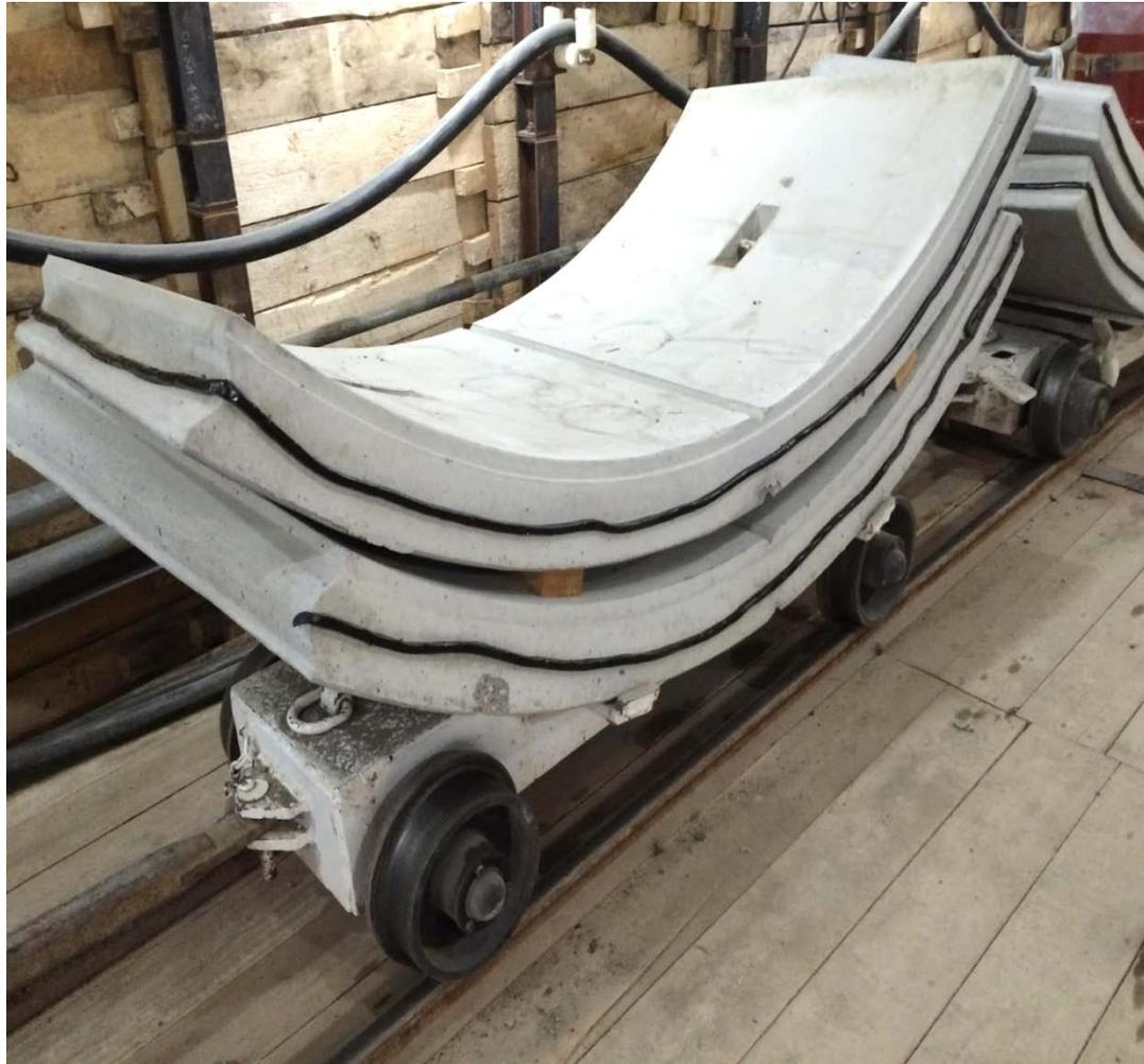
**Figure 1g: SESS Stage SW4- Pre-cast concrete liner segments, 2.9 m panels- Transported from working shaft to TBM using segment carrier cars**
