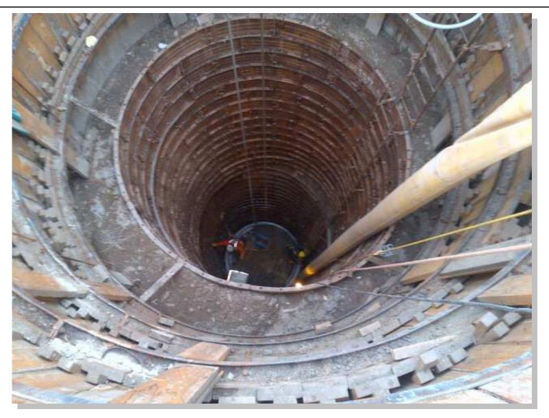
Figure 1d. NEST NL2/NL3/N1 – Construction of Access Manhole
