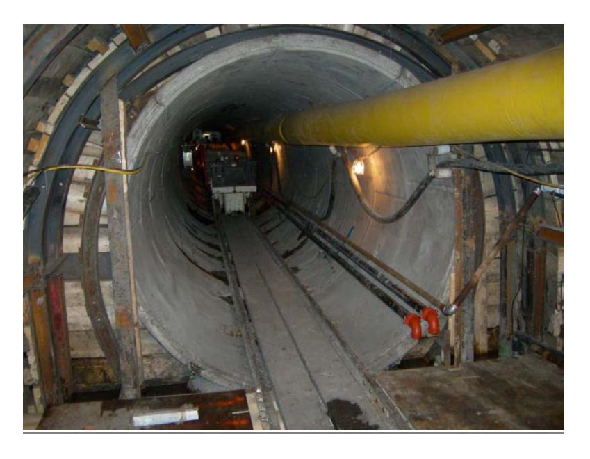
Figure 1(C) SESS (SW2/3) – Tunnel Finished with Concrete Liners
