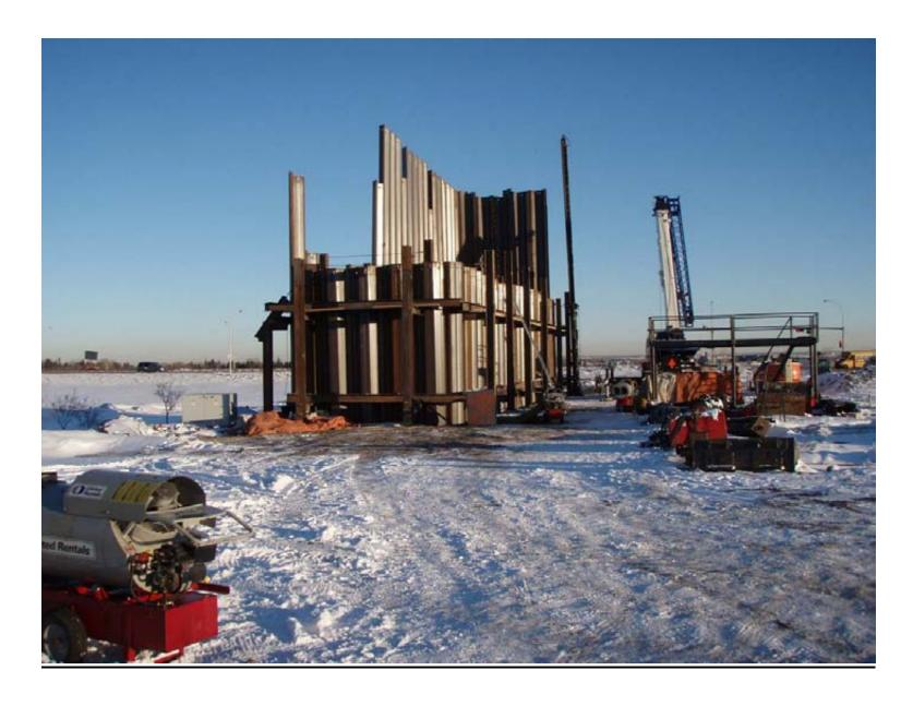
Figure 1(f) NEST (NL2/3&N1) – Working Shaft Commenced With Sheet Piling
