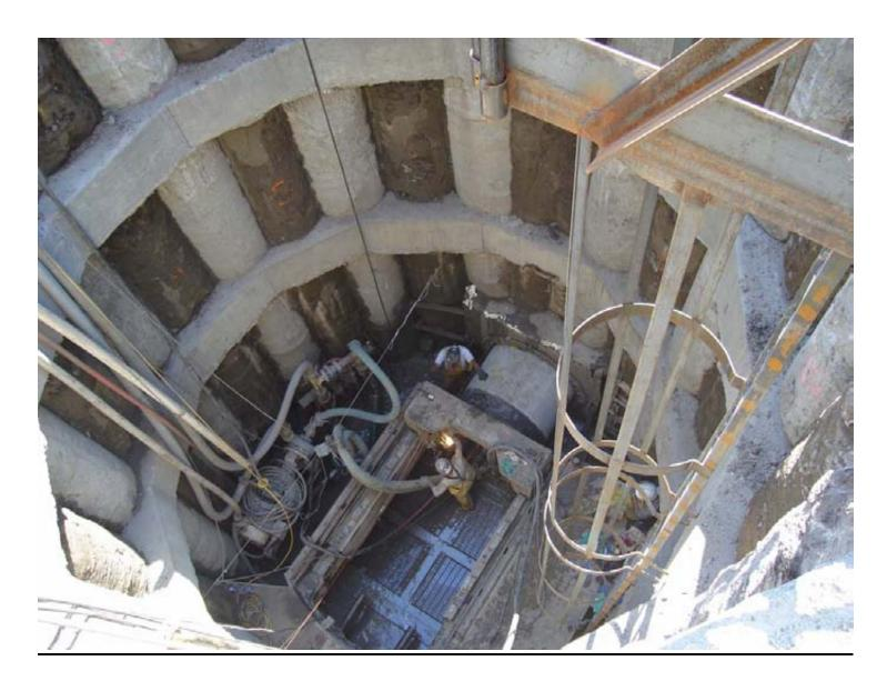
Figure 1(d)-WESS (W1) – Microtunnelling in Progress
