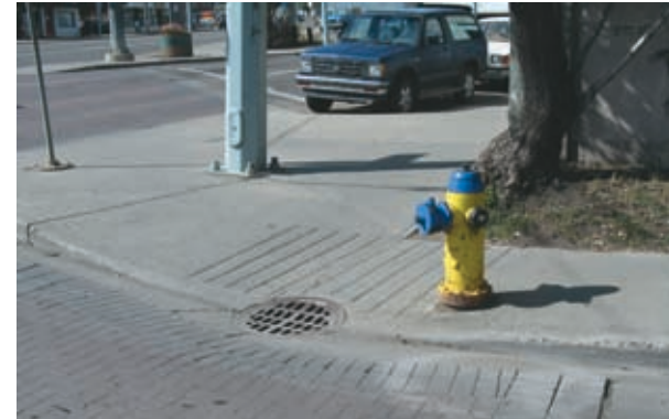
Existing utility services
