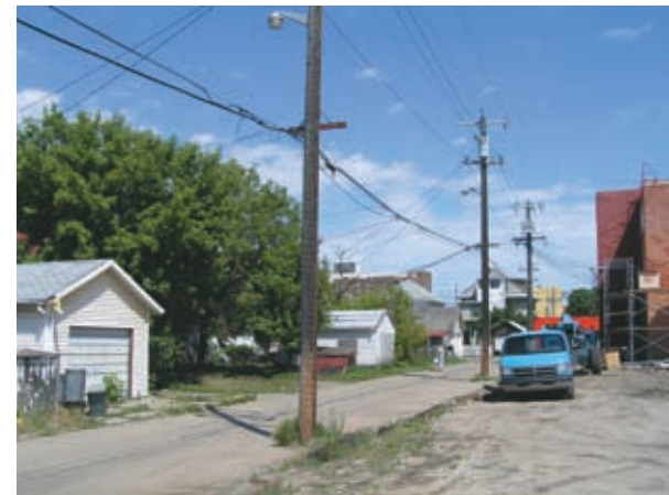
Existing utility services
