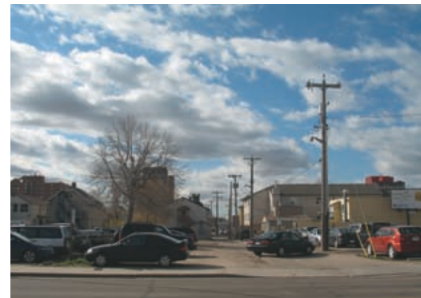
Overhead wires along laneway of 96 Street
