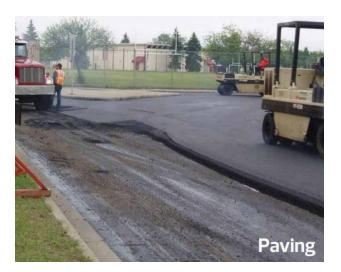
Paving is the quickest step. Contractors can usually pave 3–5 blocks per day.
