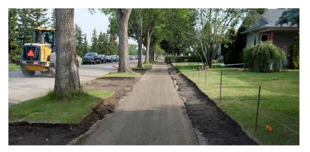
Forms are set in order to pour new concrete for the sidewalk.
