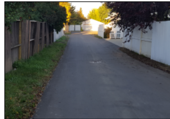
After alley renewal
