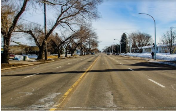
Existing condition at 132 Avenue near 122 Street. Two lanes of traffic in each direction, with a parking lane on the south side.
