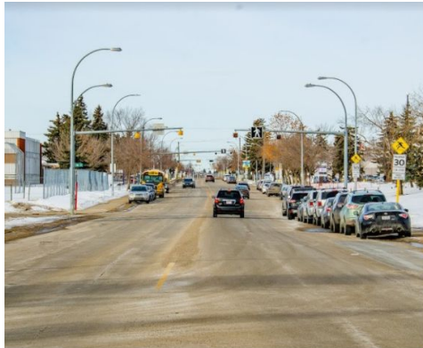
Existing conditions at 132 Avenue near 86 Street. One lane of traffic in each direction with a parking lane in each direction
