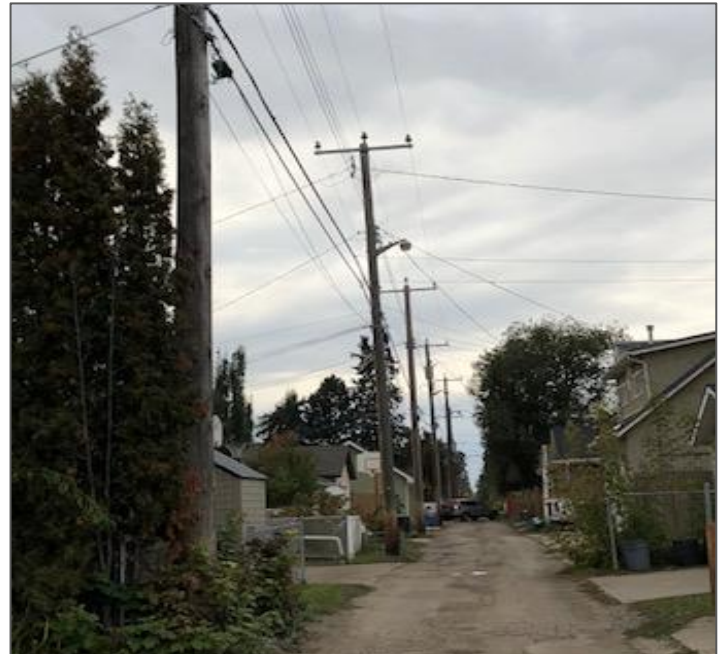
Alley with existing poles
