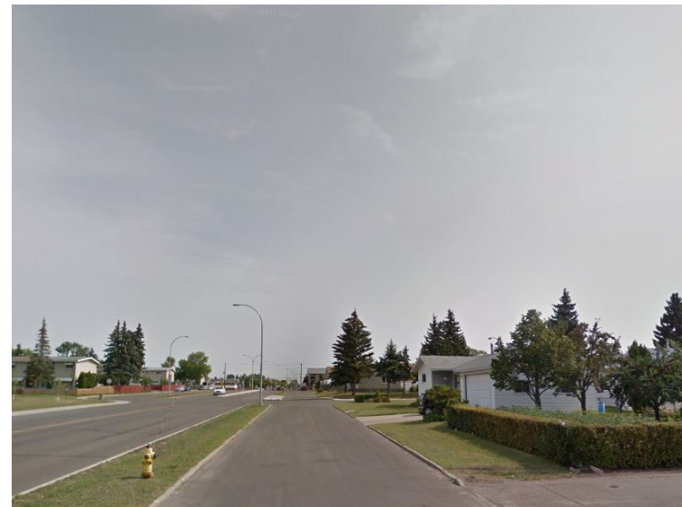
Figure 25. 132 Avenue service road looking east
