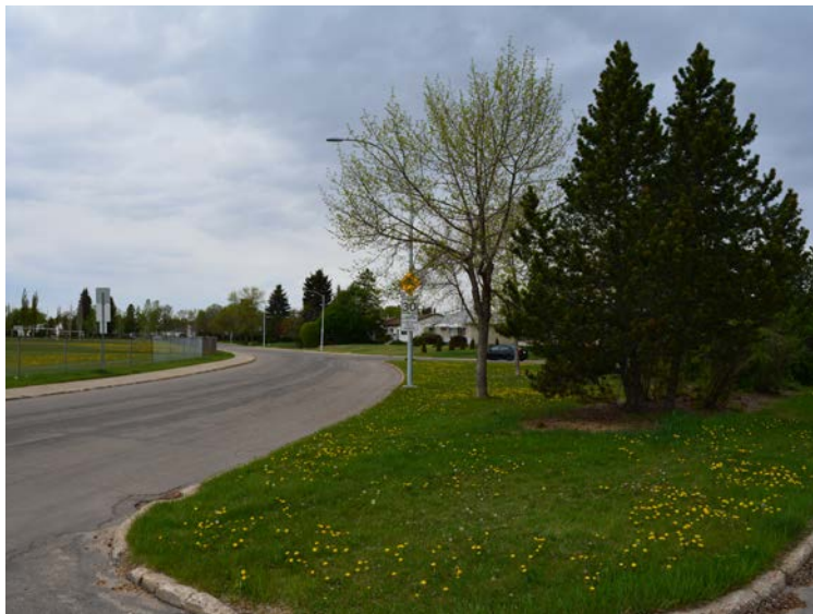
Figure 5. 129B Avenue roadway green space existing conditions
