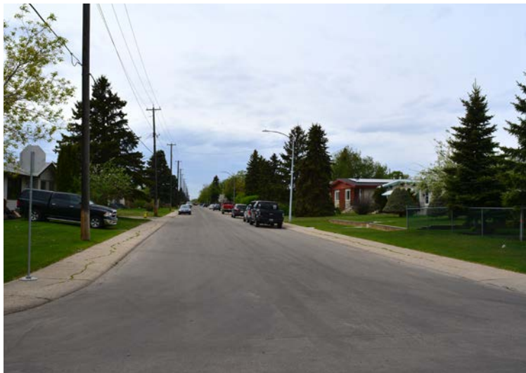
Figure 20. 128 Avenue looking west at 92 Street
