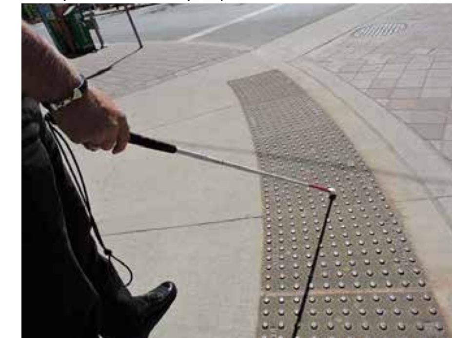
Tactile Walking Surface Indicators Used at intersection curb ramps to improve safety for the visually impaired.
