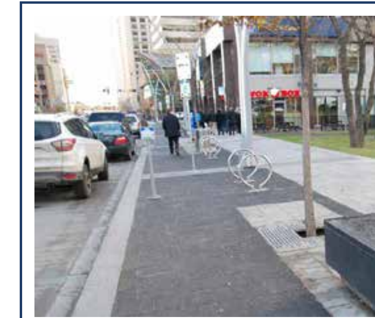
High-Contrast Furnishing Zone Surface Contrasting colour of paving in the furnishing zone improves wayfinding clarity for the visually impaired. Dark colour concrete paving stones, similar to Jasper Avenue New Vision are proposed.
