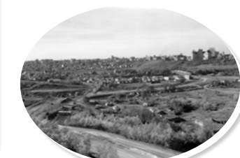
View of Low Level Bridge, Connors Road and Future Gallagher Park Site [EA-600-5027a]
