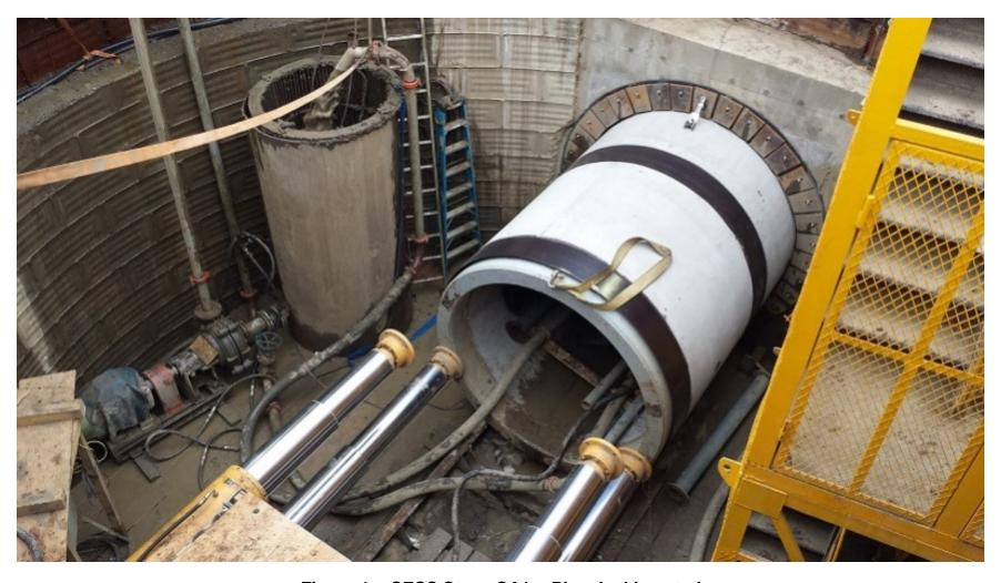
Figure 1a: SESS Stage SA1a- Pipe Jacking station
