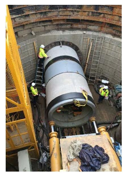
Figure 4. SESS SA1a – Pipe Jacking station in the working shaft at MH 103
