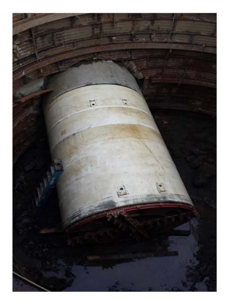
Figure 3. SESS SA1a- TBM head breaking through the receiving shaft at MH 102
