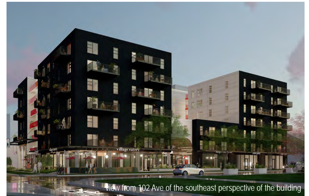
view of the 102 Ave commercial pedestrian interface
