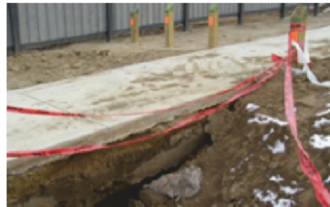
Undermined sidewalk
