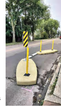
Adaptable curb extension on 102 Street and 82 Avenue, as part of the Ritchie Street Lab.
