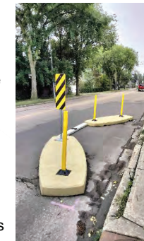
Adaptable curb extension on 102 Street and 82 Avenue, as part of the Ritchie Street Lab.
