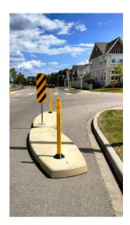
Adaptable curb extensions will be added in some locations. Adaptable curb extensions extend into the roadway, either at crossings or mid-block and help to define the use of the road. They are typically placed to provide shorter crossing distances near pedestrian crossings or to help define where parking is permitted.
