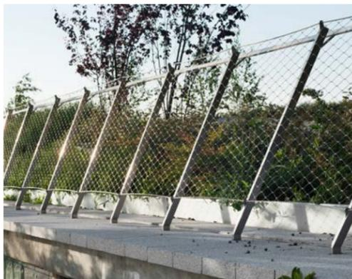
GALVANIZED HANDRAILS WITH MESH INFILL
