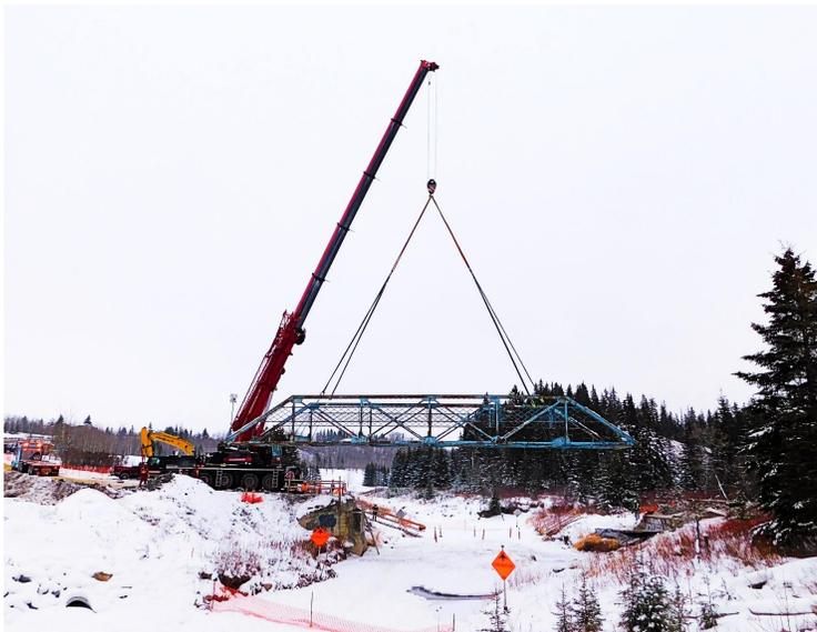
During the winter, work also focused on installing the bridge foundations and preparing the site for the new bridge. The abutments (concrete structures that support the bridge) are currently being finished and earthworks will continue through the spring. Meanwhile, the steel bridge truss structure is being fabricated off-site. Once the truss structure is complete, it will be raised into place on the abutments before the concrete deck is poured.
