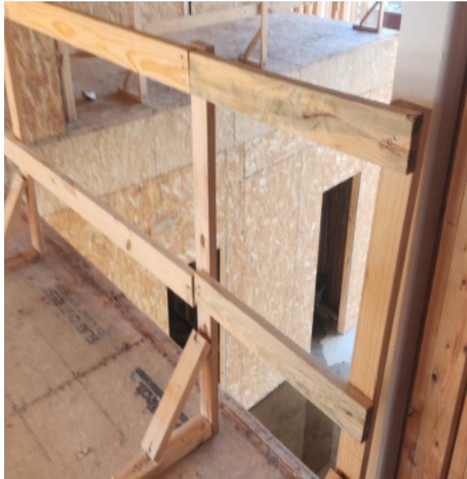
Secure guardrail installed to prevent fall hazards.
