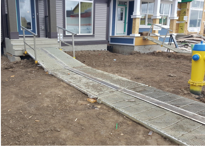
Solid supports and handrail in place for safe access.
