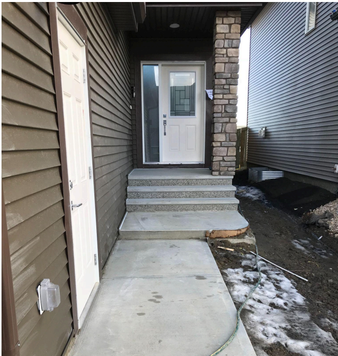
Wide stairs and 3 risers so handrails are not required.
