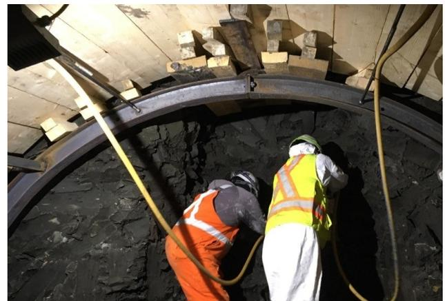
Figure 1b - NEST NC2/NC3, Undercut Excavation
