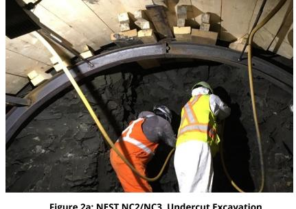
Figure 2a: NEST NC2/NC3, Undercut Excavation
