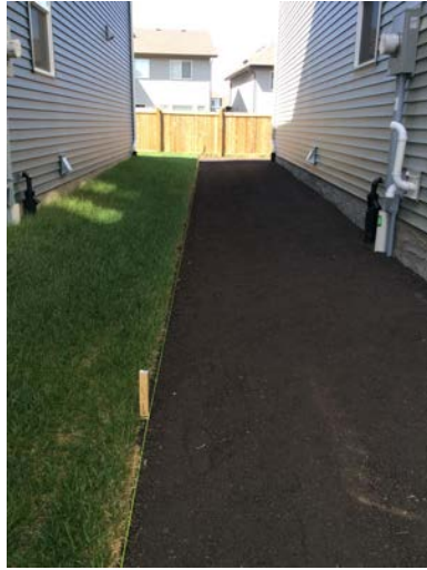
Figure 7 - Common Property Line Swale
