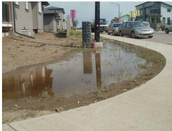
Figure 16 - Example of clay cap at Rough Grade
