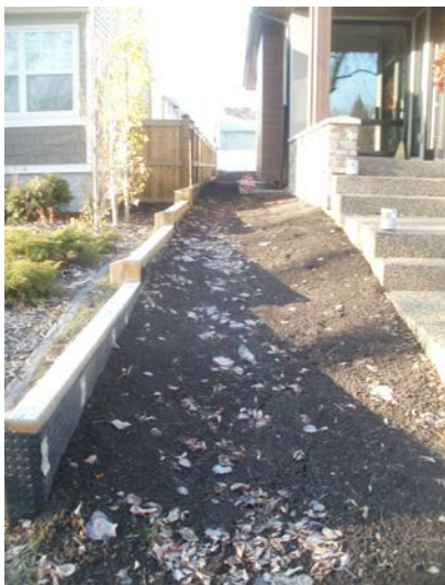
Figure 10 - Wooden retaining wall
