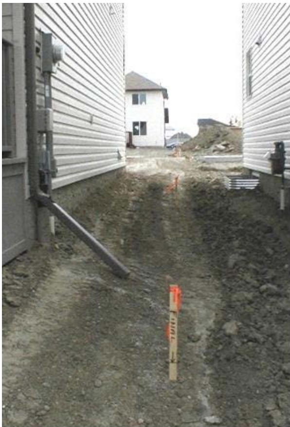
Figure 1 - Example of Rough Grade
