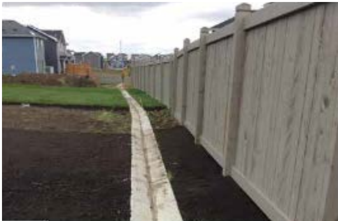
Figure 17 - Major concrete drainage swale easement
