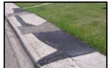
Asphalt patching
