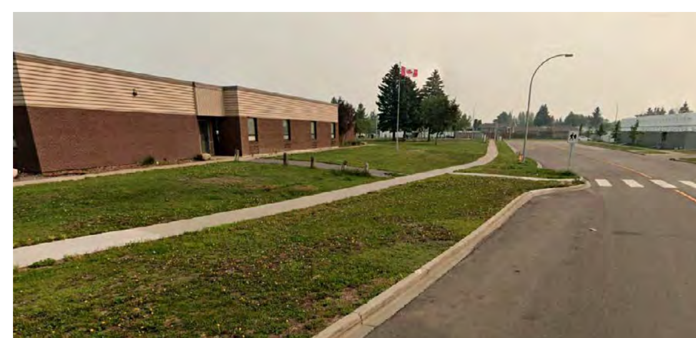
Photo of Existing St. Maria Goretti School Drop off
