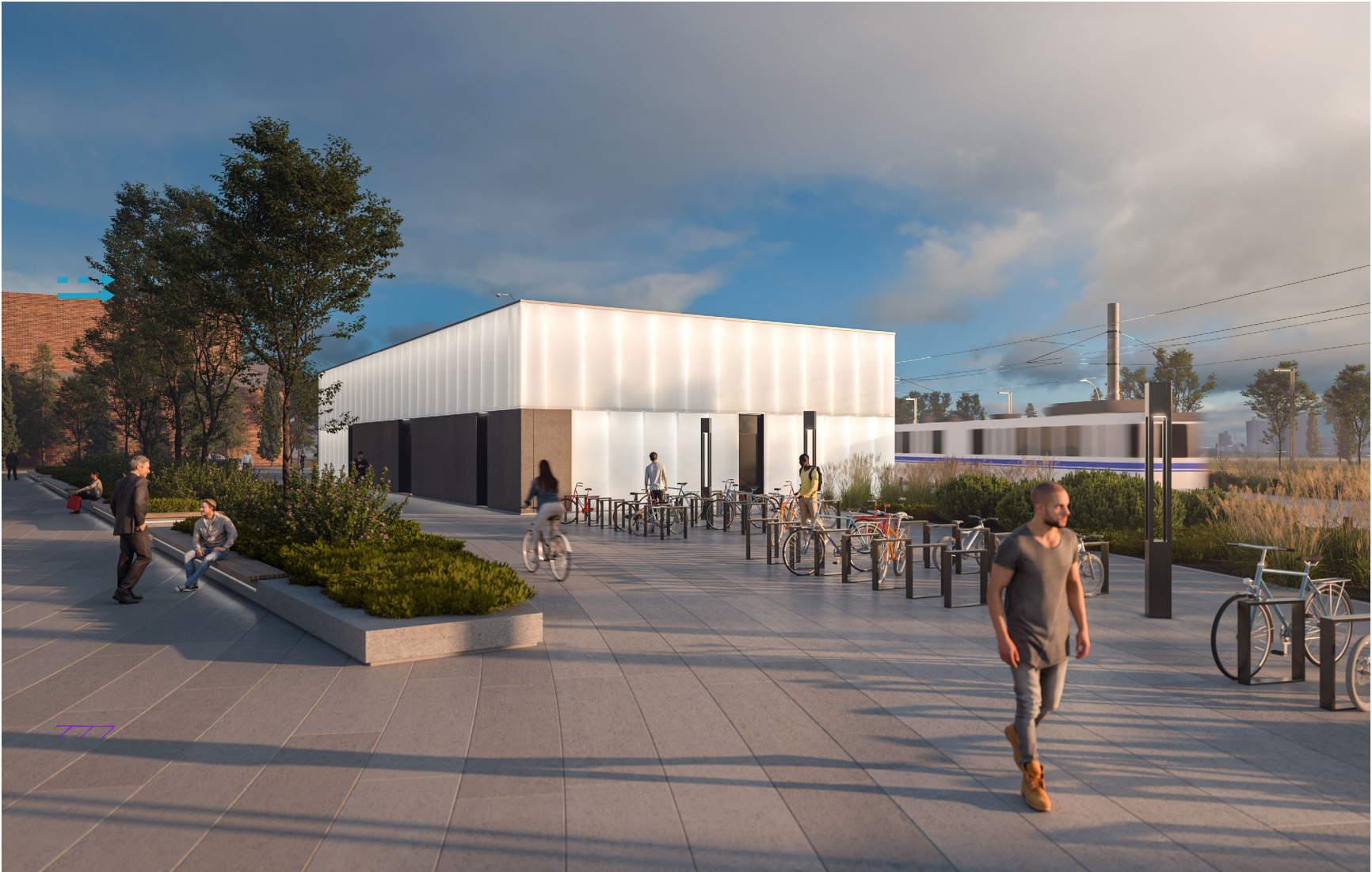
This utility complex stores equipment to power the LRT system. It features LED-backlit glass panels, making it a prominent feature in the new NAIT/Blatchford Market plaza.
