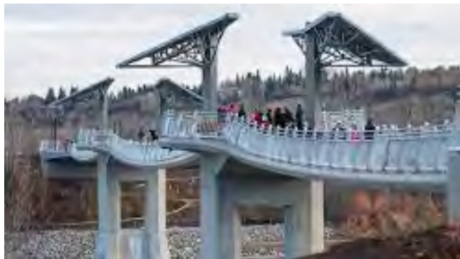
Terwillegar Park Footbridge
