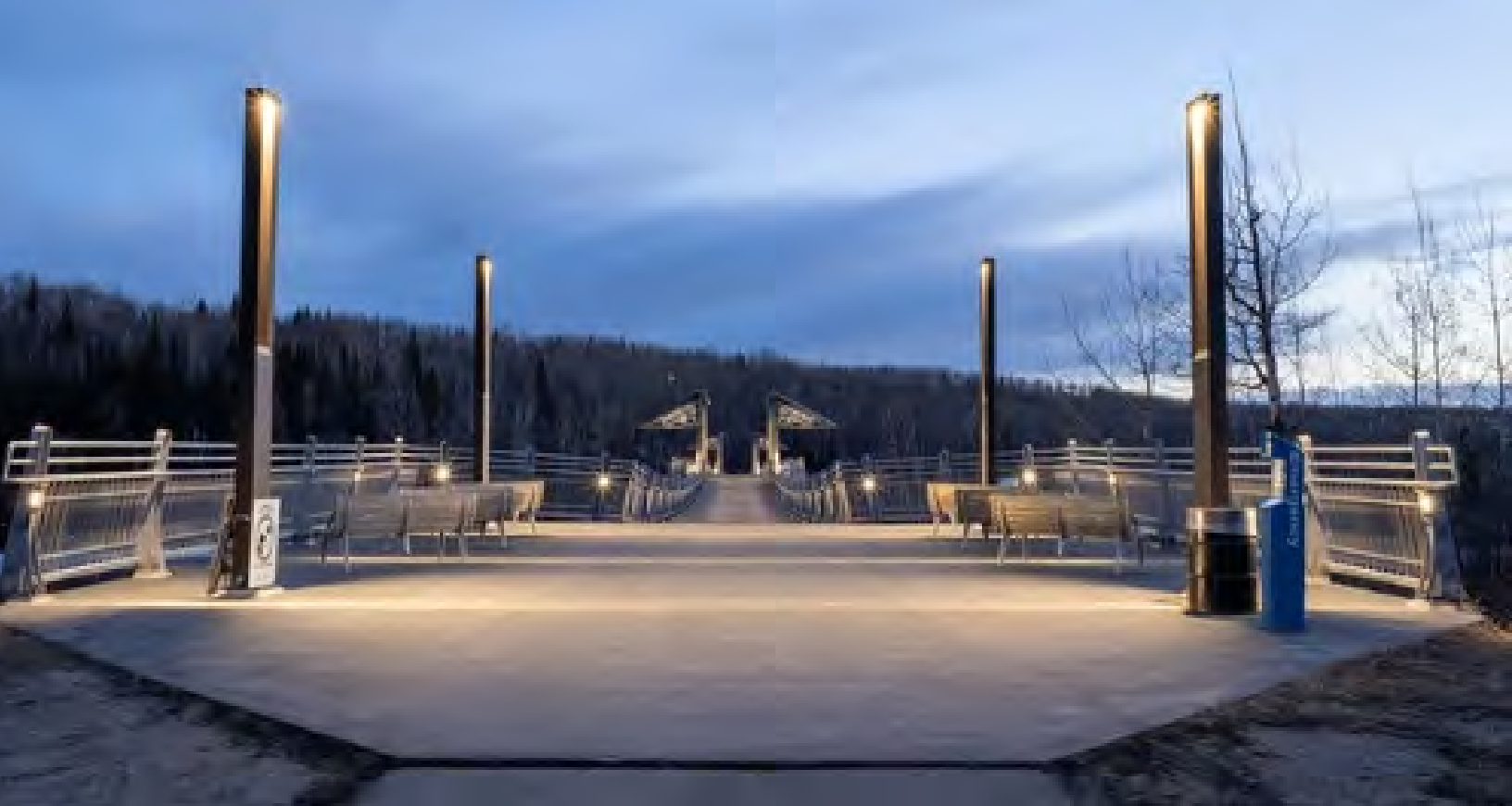
Approach to Terwillegar Park Footbridge from Jan Reimer Park
