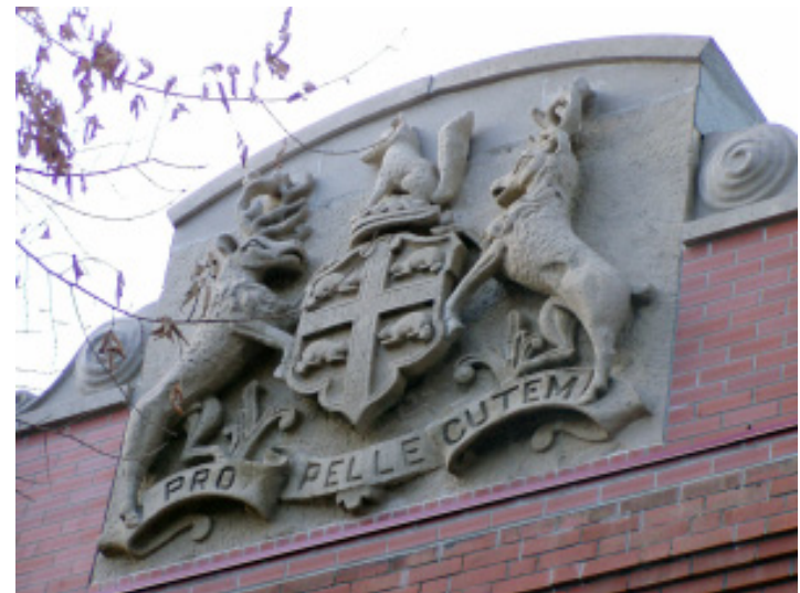
Ortona Armoury detail
