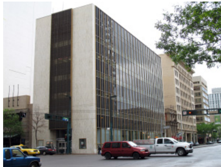
TD Bank Building on Jasper Avenue
