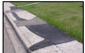
Asphalt patching
