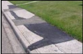
Asphalt patching
