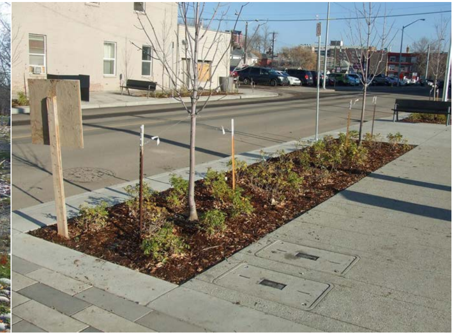
FIGURE 36 - TREES IN STRUCTURAL SOIL CELLS
