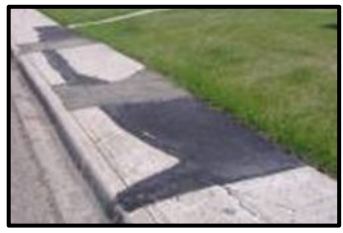
Asphalt patching
