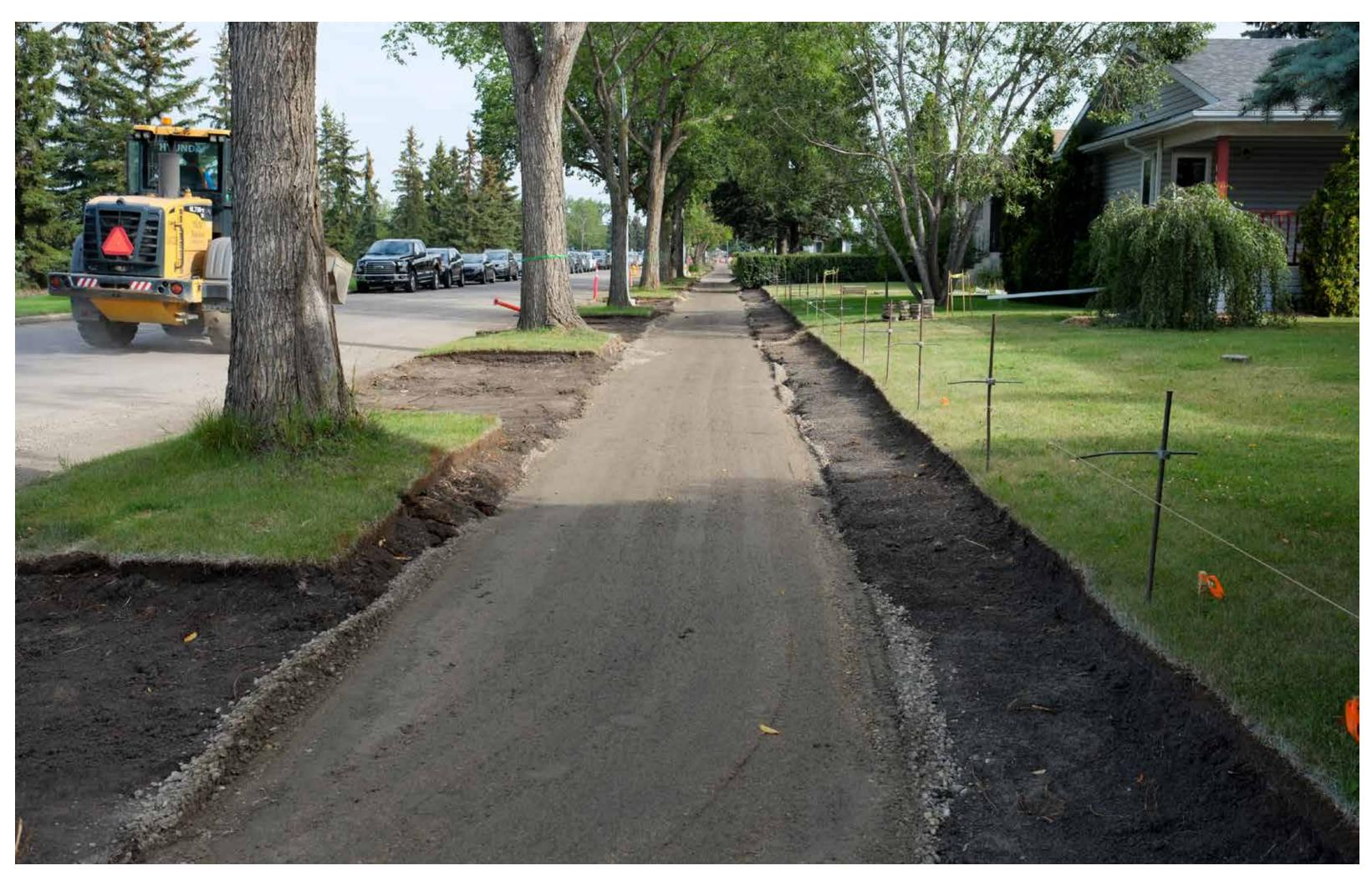
After removal of the existing sidewalk, gravel is placed and compacted to prepare for construction.
