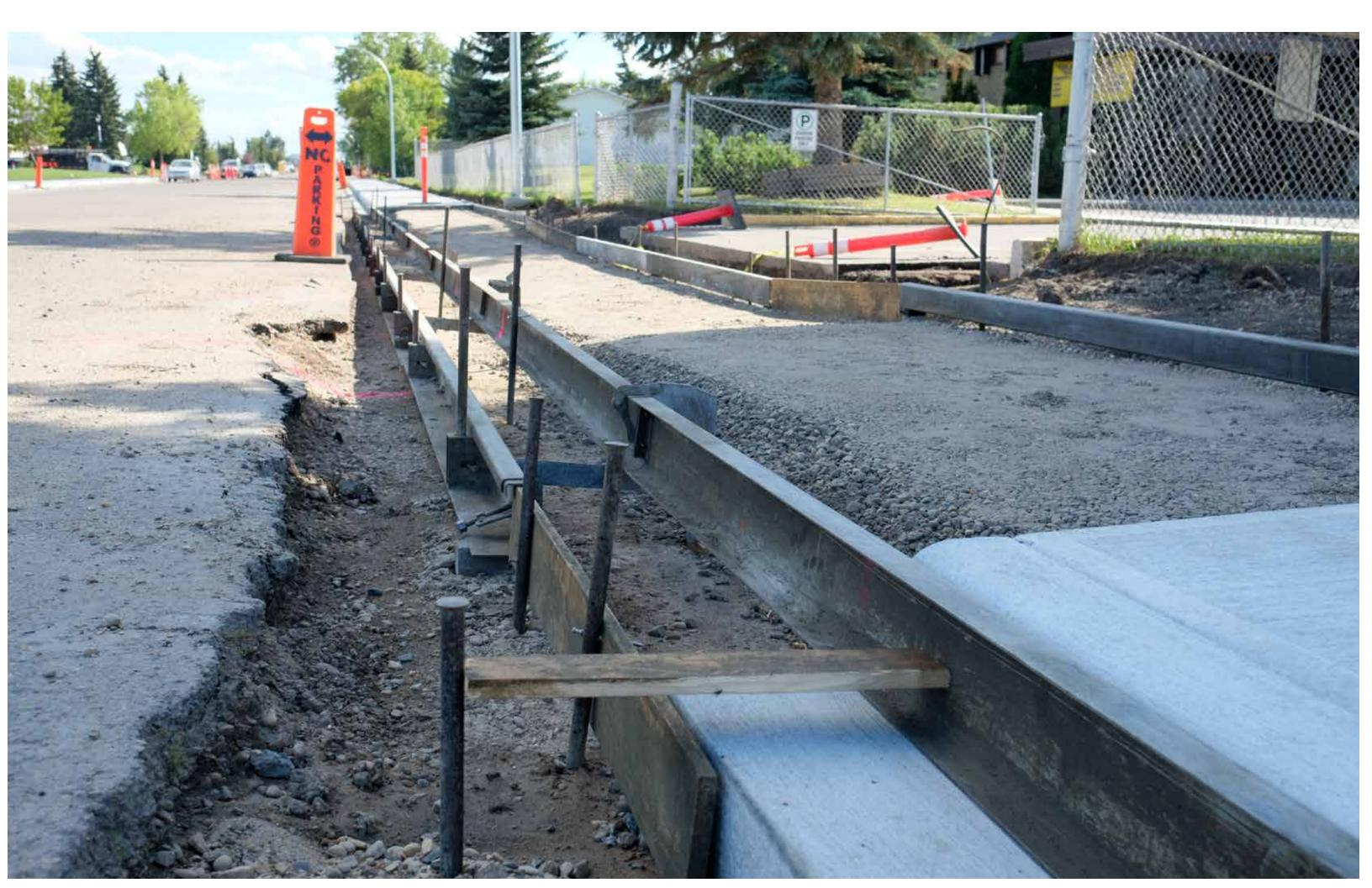
Forms are set in order to pour new concrete for the sidewalk.
