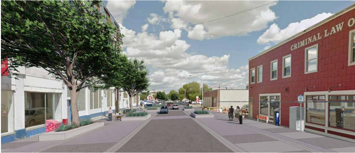
103 Avenue looking east from 97 Street
