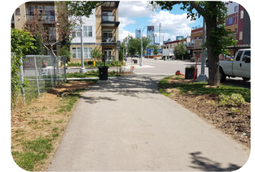
Typical boulevard-style shared pathway
