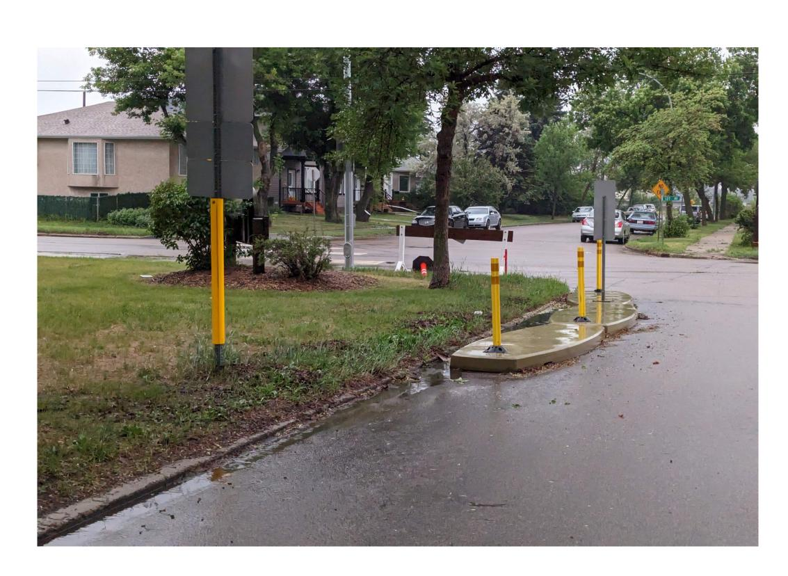
Oval-shaped precast slabs of concrete typically located along curb edge of a roadway to narrow traffic lanes to slow vehicles and outline parking areas. They are currently used in Edmonton, St. Albert and Calgary.
