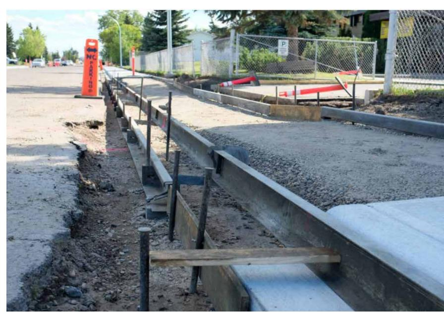
If a sidewalk is machine poured, a stringline is used to set grades as it pours the concrete.
