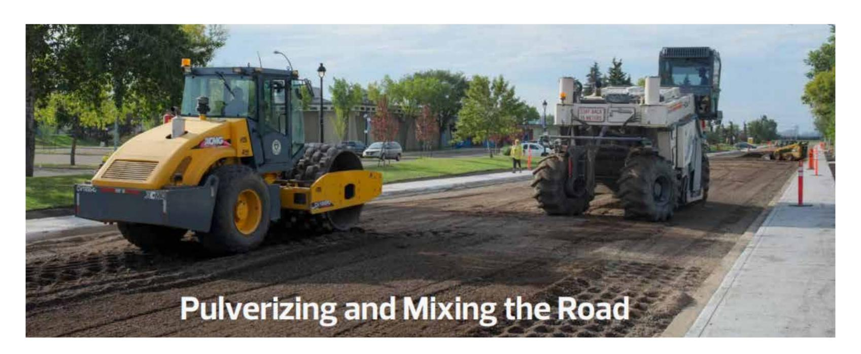
The graded road base needs two to three days for it to cure prior to paving and can be driven on. The road will be fully closed during paving operations and typically opens later on the same day.
