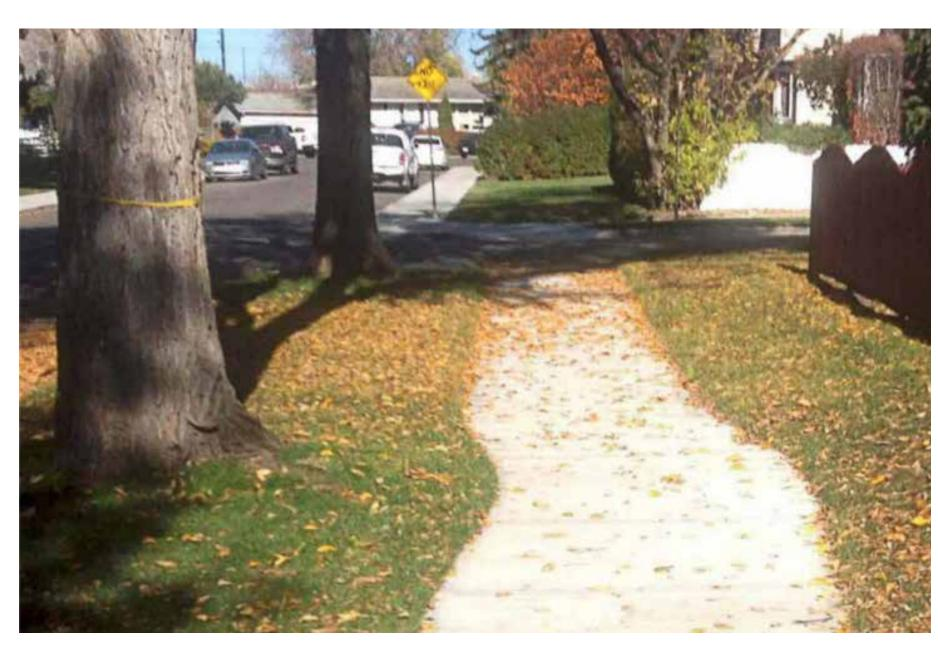
Extra deep cuts and rebar are added to the sidewalk to control where it may crack and to keep the sidewalk intact as the tree's roots grow.
