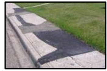
Asphalt patching
