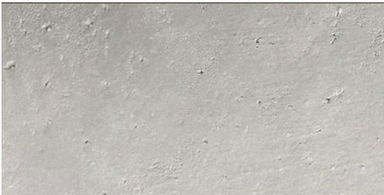
3 - ARCHITECTURAL FINISH CONCRETE
