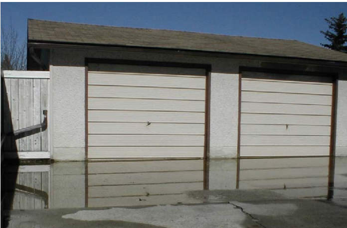
Low areas in the yard can result in pooling and flooding during heavy rain or snow melt
