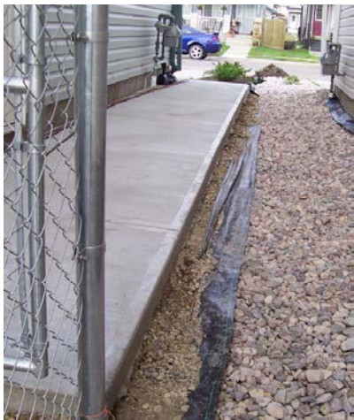
This new sidewalk does not have 15 cm drainage space within the property
