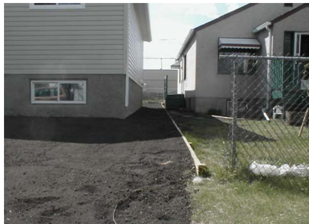
Internal swales for an infill house adjacent to properties with existing grade sloping towards the foundation walls.
