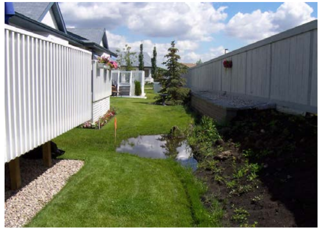
Poor grading in this drainage swale causes water pooling
