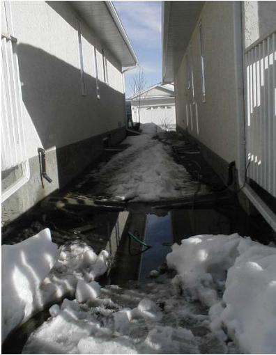
Poor lot grading results in flooding between two condominium units
