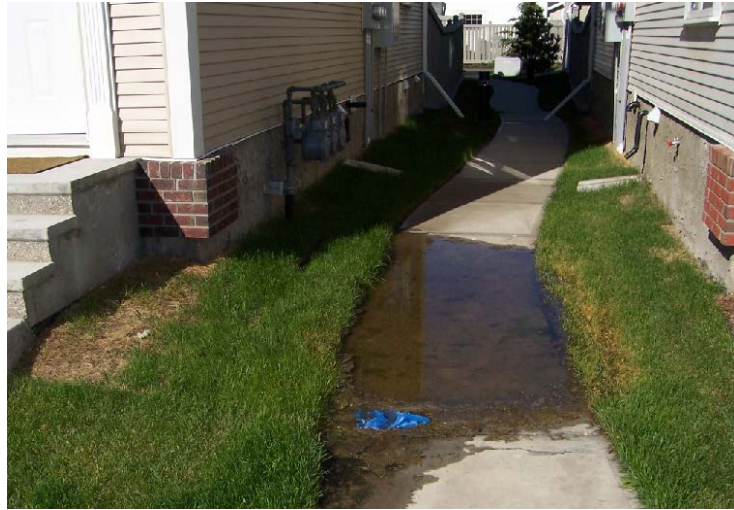
Sidewalk settlement between two condominium units results in pooling of water
