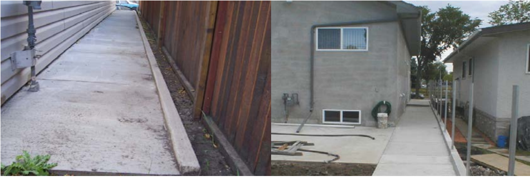
These new sidewalks, with raised edges, create internal swales which prevents surface water drainage towards the adjacent lots
