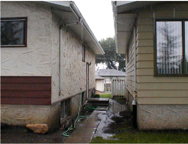
Areas with poor lot grading generate a risk of basement flooding during rain events
