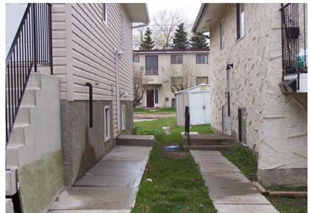
Sump pump discharge on the left drains towards the right property which has a slope towards the foundation wall
