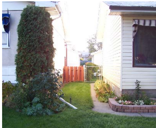
This downspout directs stormwater towards a neighbour's lot which has a slope towards the foundation wall
