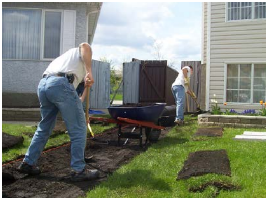
An internal drainage swale is being built with a string-line as a visual guide for the slope of the swale
