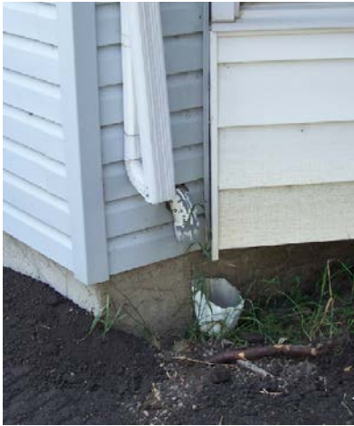
Downspout disconnected from storm service
