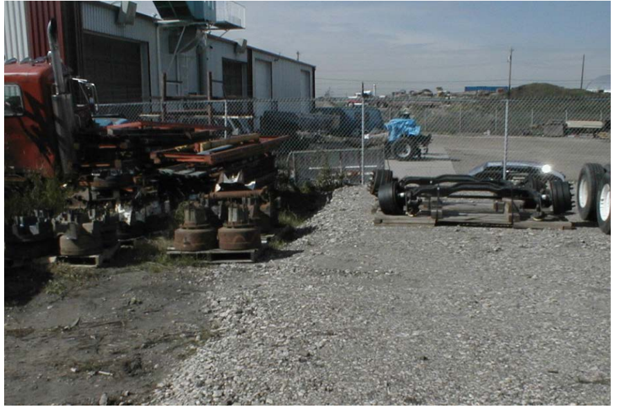
This new industrial development has no on-site stormwater management. The gravel is graded high and slopes towards the existing industrial site behind the fence.
