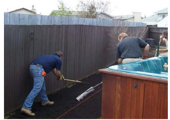
An internal drainage swale is being built with a string-line as a visual guide for the slope of the swale
