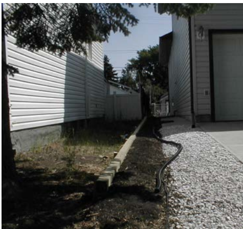
Internal swales for an infill house adjacent to properties with existing grade sloping towards the foundation walls.
