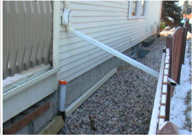
Downspout disconnected from the storm service and directed towards the neighbour's property is a violation of the Bylaw
