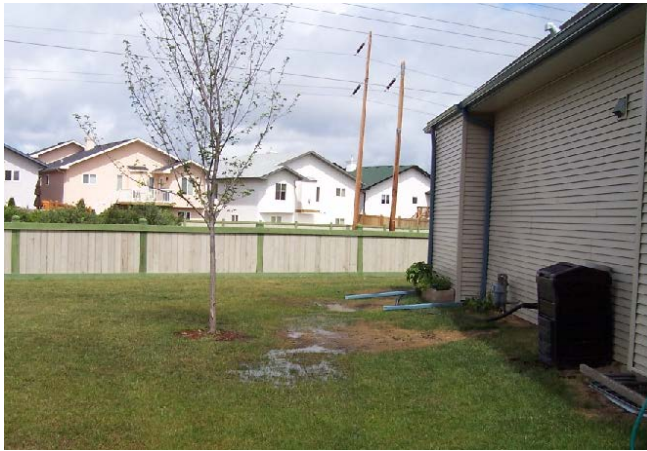
Settlement beside this condominium unit causes water pooling and potential basement flooding
