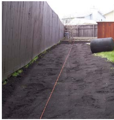
An internal drainage swale is being built with a string-line as a visual guide for the slope of the swale
