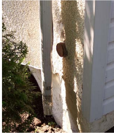
Downspout disconnected from storm service which drains into a pipe that runs between the floor joists
