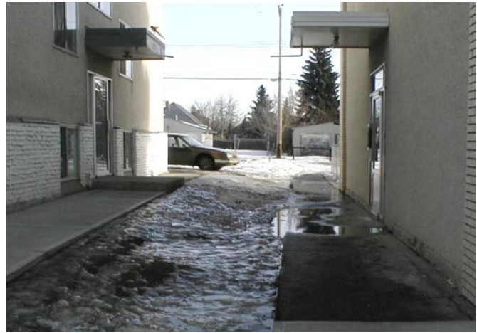
Poor lot grading between two apartments creates a low area for ponding during snow melt
