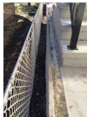
Concrete internal swale adjacent to concrete sidewalk
