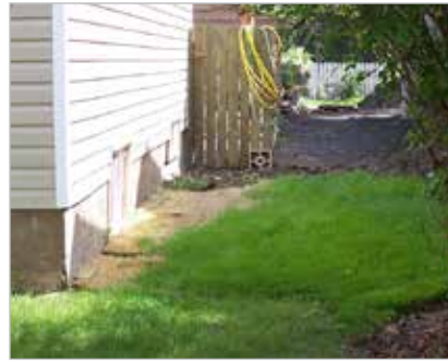
A lot that is regraded without creating a common or internal drainage swale will direct stormwater to an abutting property with negative grade.
