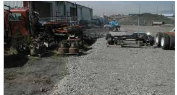
The new industrial development has no on-site stormwater management. The gravel is graded high and slopes towards the existing industrial site behind the fence.
