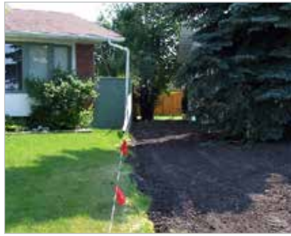
A lot that is regraded without creating a common or internal drainage swale will direct stormwater to an abutting property with negative grade.
