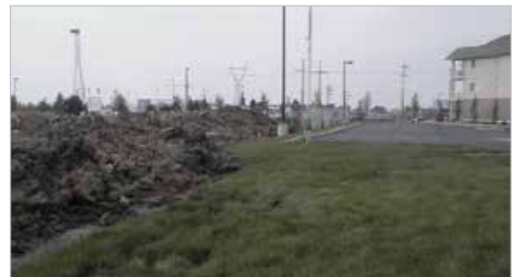
This new apartment site is in violation of the bylaw because it has the surface runoff flowing towards the abutting lot.
