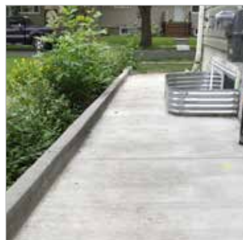
Example of a sidewalk with a curb/retaining wall to create an internal swale
