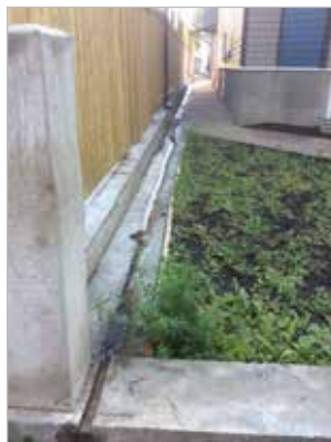
Concrete retaining wall and internal swale
