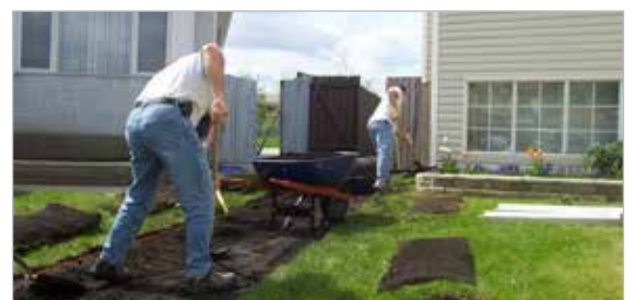
An internal drainage swale being built using a string-line as a visual guide for the slope of the swale
