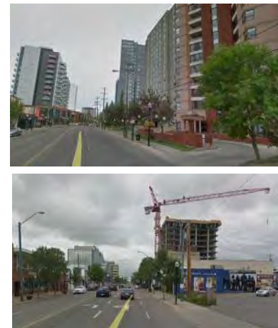
Image 5: Street views from the intersection of Jasper Ave and 124 St NW to the east (upper) and north (lower) (Courtesy of Google Earth)
