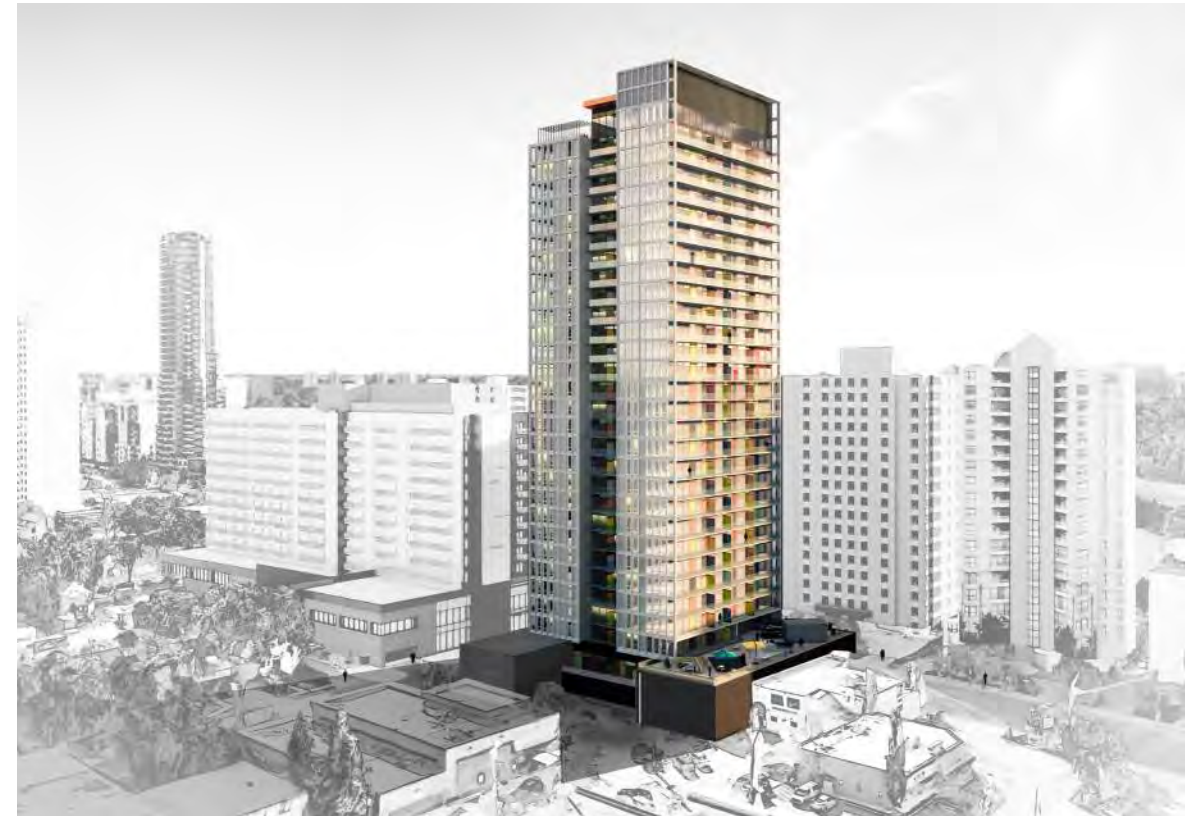
View of the tower and podium looking southeast
