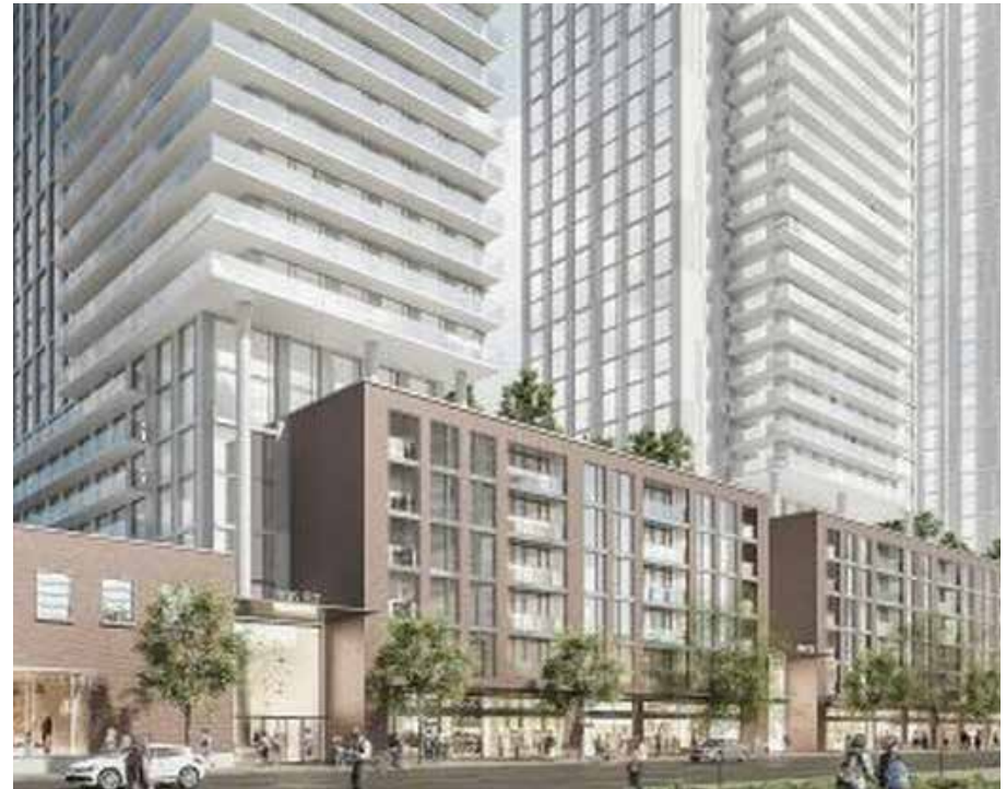
Located on 106 Street NW and 103 Avenue NW, the Massey Ferguson Building Redevelopment is a residential, office and retail building in its pre-construction stage. There are a total of three buildings of 48, 45 and 42 storeys with a total of 1300 units.
