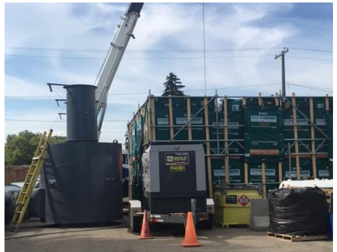
Noise barriers around the pump station at 151 Street and 99 Avenue
