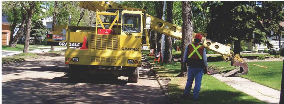
▲ Removing old sidewalk for sidewalk renewal.
