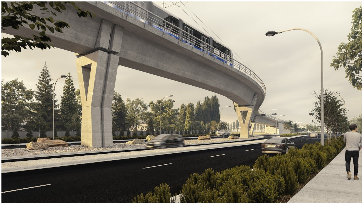
Future 87 Avenue Elevated Guideway
